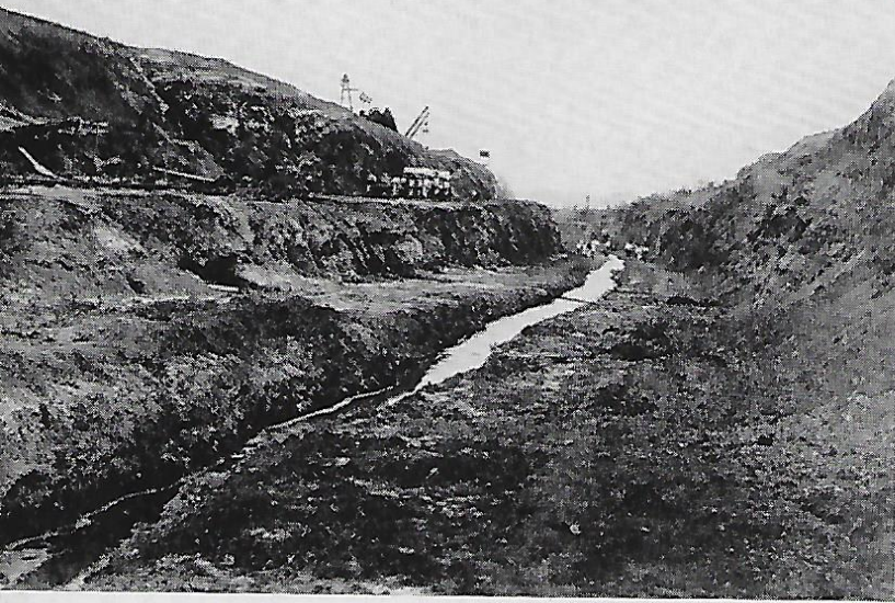
These old pictures, taken at Culebra Cut between 1896 and 1898, indicate the amount of progress made by
