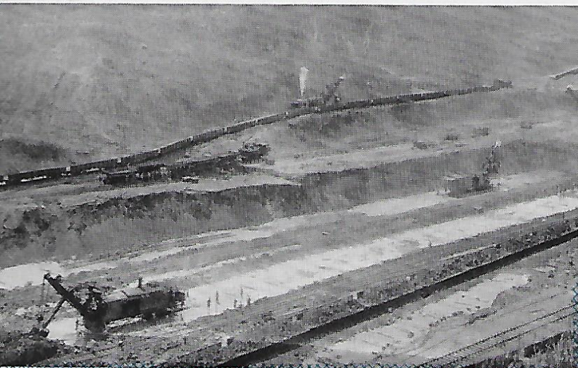
American builders used powerful steam-shovels and railroad techniques to move entire mountains of earth..
